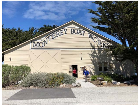
Monterey Boatworks Building (photo by Brian Palermo)
